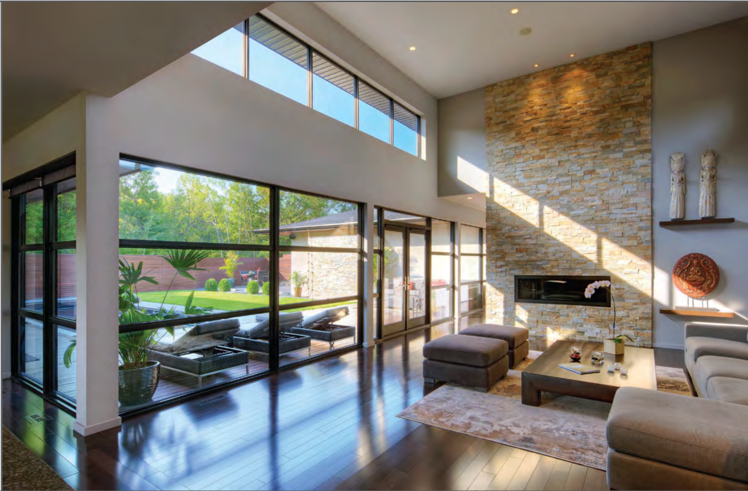
Triple pane low-E glass with insulated fiberglass frames
